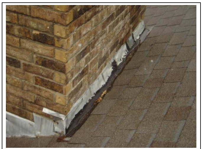
Caulking repairs around chimney flashing
